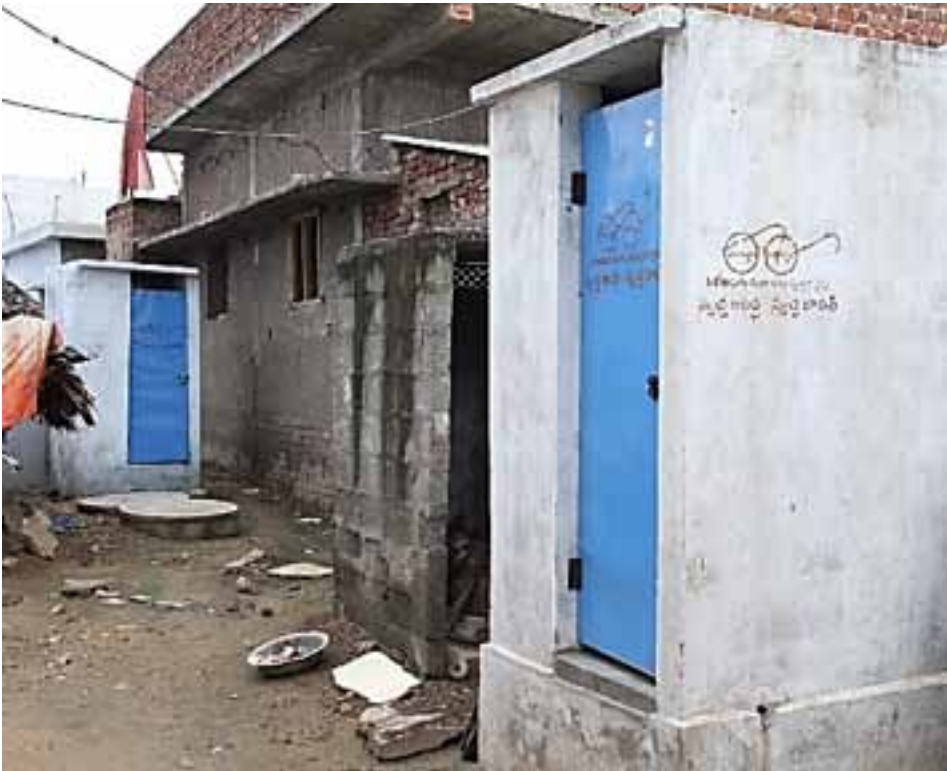
Toilets build in the ABD area in Kakinada
