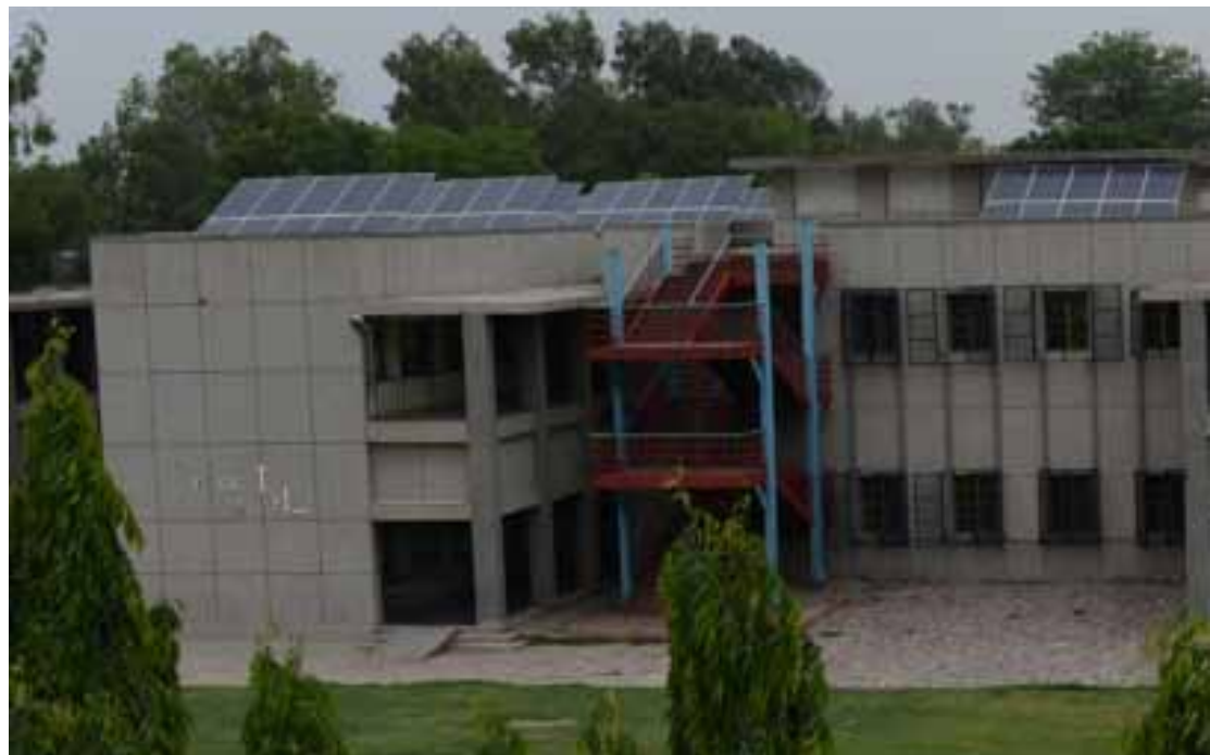
Solar Rooftop installed on a NDMC School building
