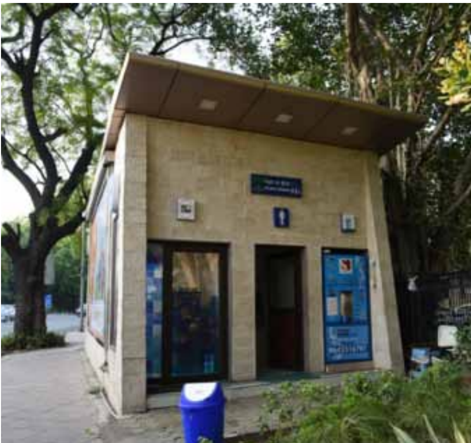
Public Toilet along with Water ATM and Bank ATM in NDMC
